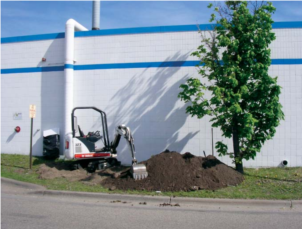
Figure 1. Excavation of insulation samples after 15 years
