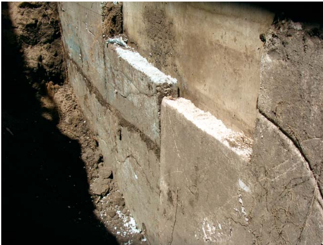
Figure 2. XPS and EPS below grade insulation
