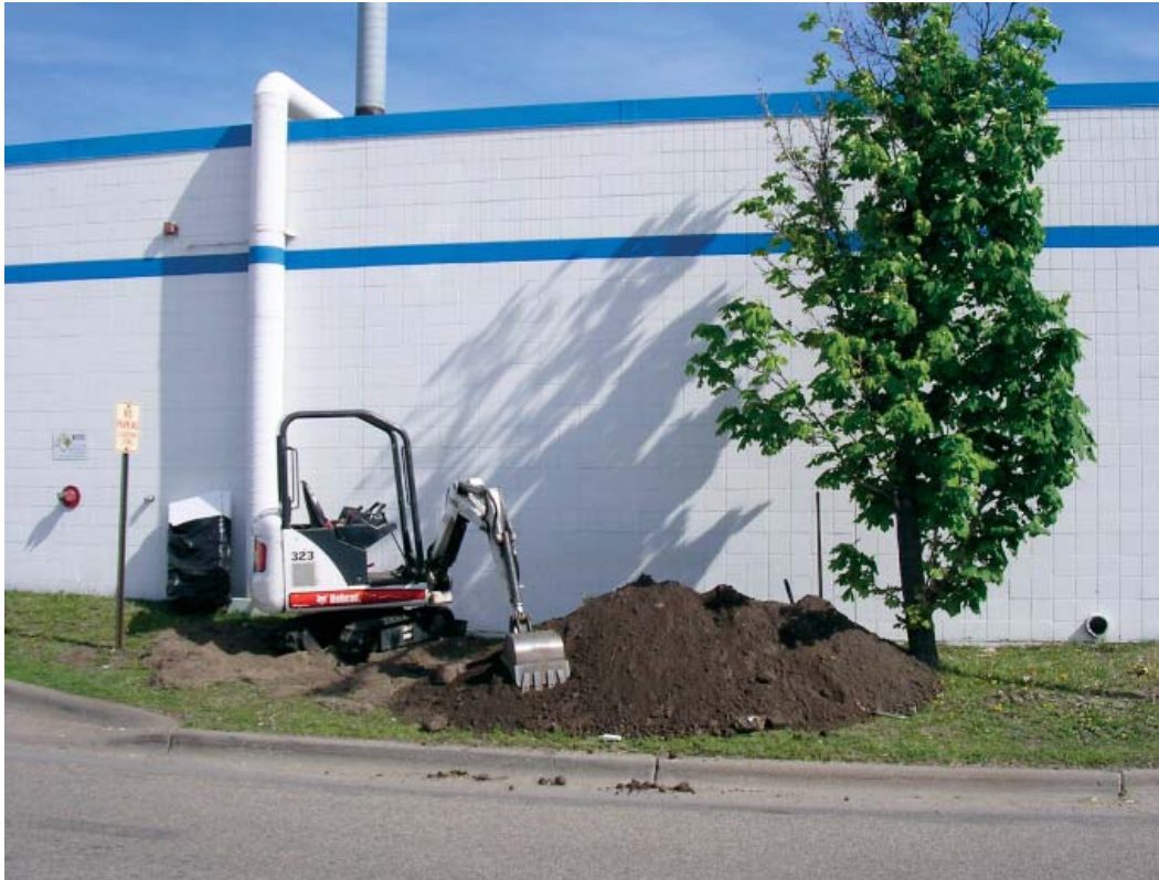
Figure 1. Excavation of insulation samples after 15 years
