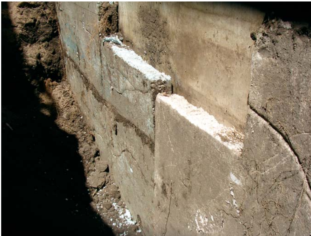
Figure 2. XPS and EPS below grade insulation
