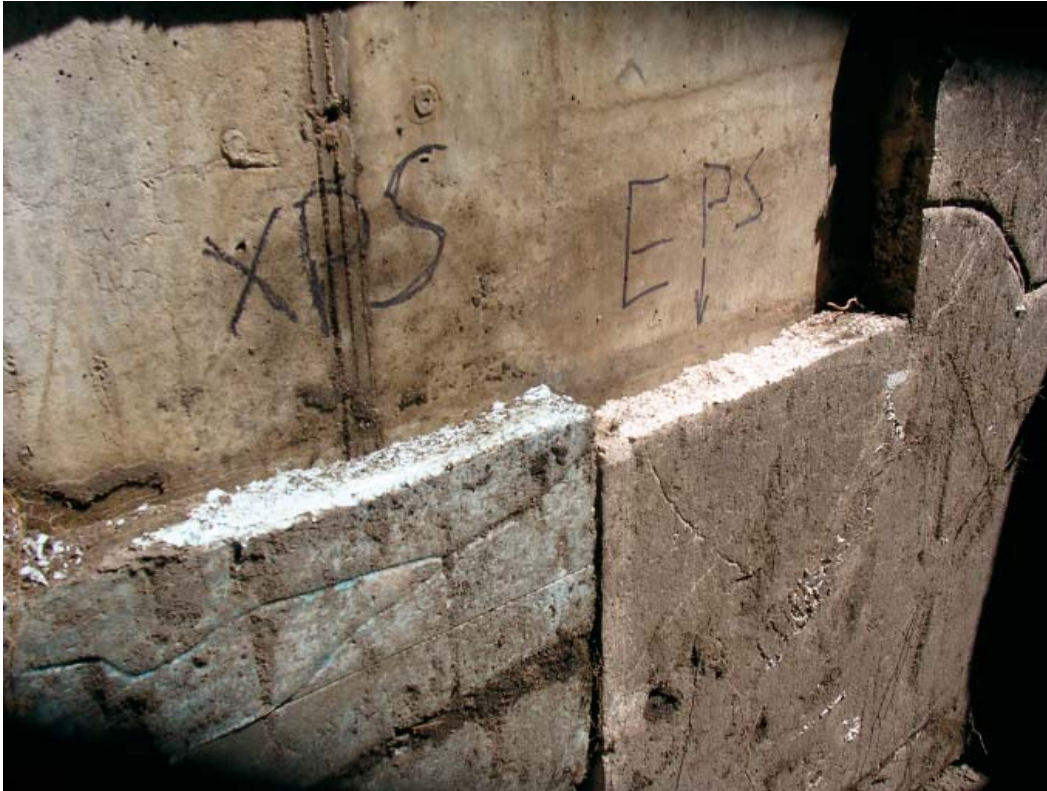
Figure 3. XPS and EPS were installed adjacent to each other
